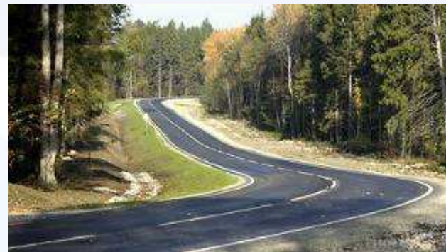
Picture: road construction, AS Aspi
